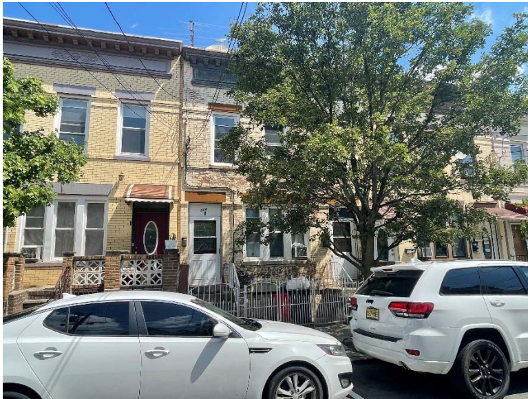
Parcel E230 (410 37, LLC) 314 14th St Union City, New Jersey
